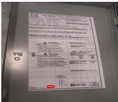
The red circle indicates the date code location inside the case of the switch
