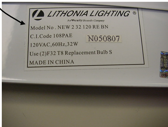
Label is inside fixture by fluorescent tube
